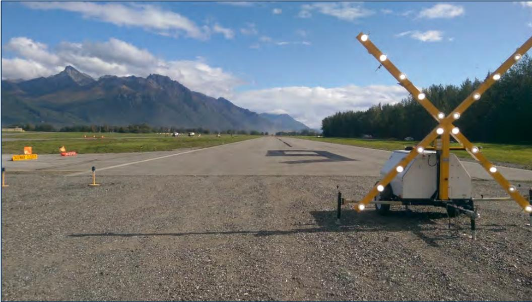
Runway 9/27 markings were removed (top photo) and remarked as runway 10/28 (bottom photo) to match the current magnetic declination.
