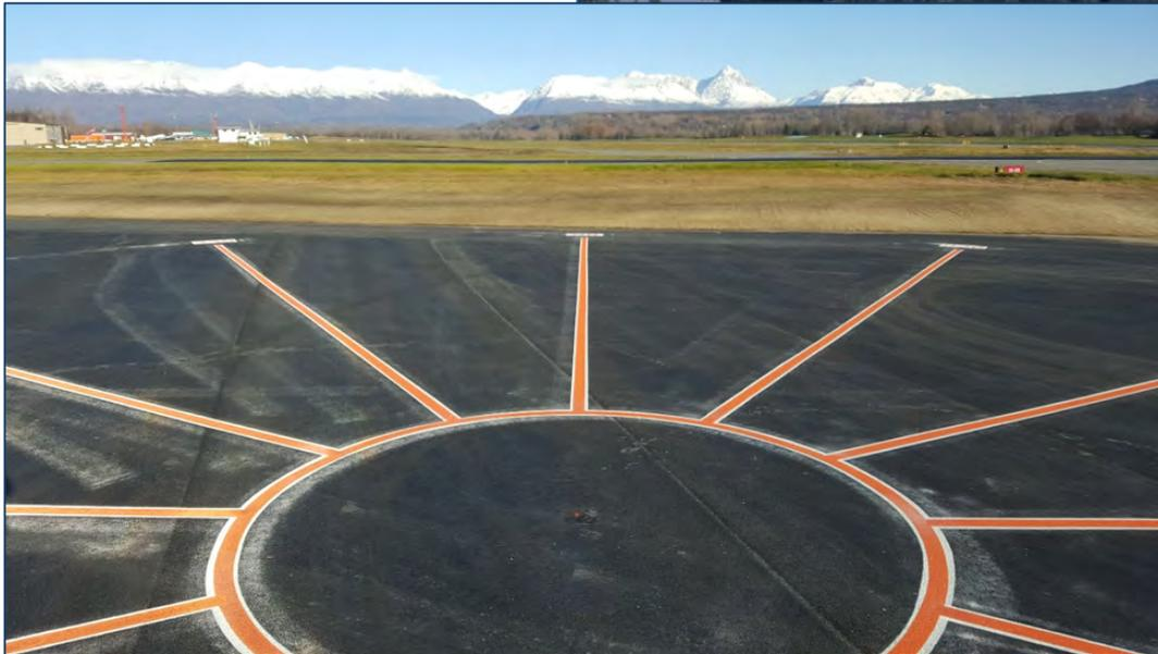
The new FAA-standard compass calibration pad on the expanded large-aircraft apron.
