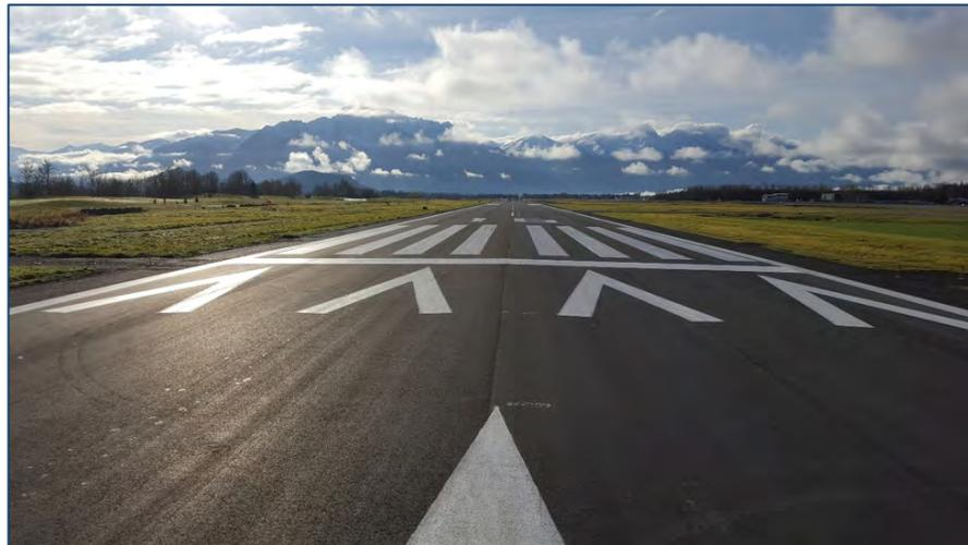
Photo: New pavement, markings, and recycled asphalt shoulders on runway 16.
