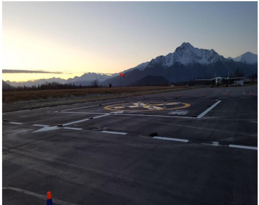
Photo: New Helipad under construction and waiting for in-pavement lighting to be installed
