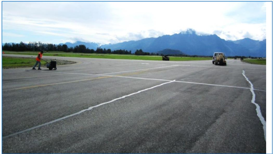
Photo: Crack sealing operations.
