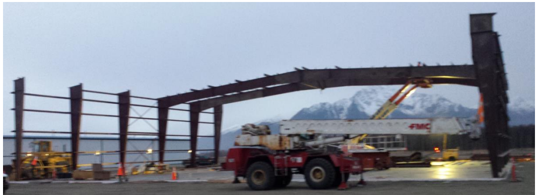
(Photo: Steppers Construction crew progresses with the roof structure)
