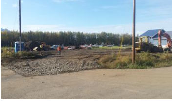
(Photo: Site work is underway in late Sept)
