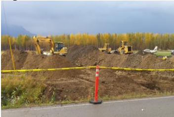
(Photo: Foundation excavation begins)
