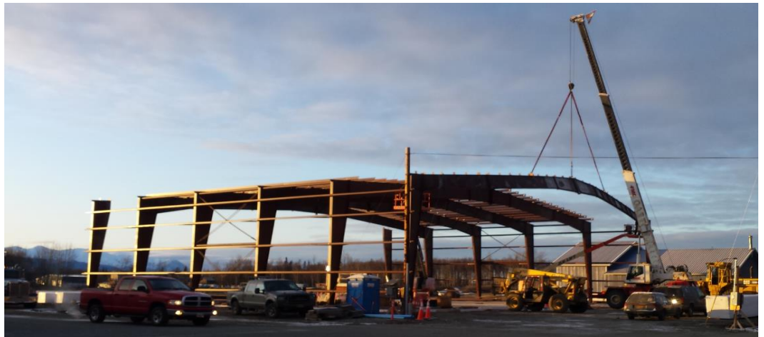
(Photo: Steppers Construction is nearing completion of the roof structure)
