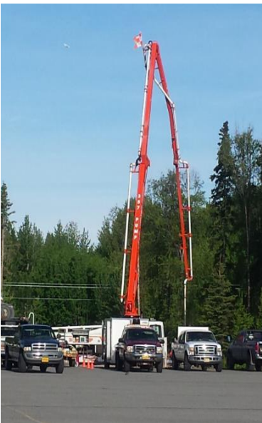
(Foundation work is completed May30th)
