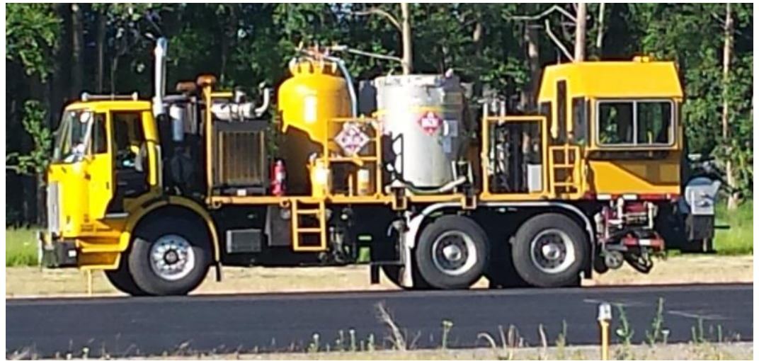
Photo: New markings being applied to runway 10/28
