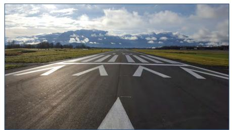
Photo: New pavement, markings, and recycled asphalt shoulders on runway 16.
