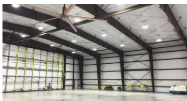
(Photo: The nearly completed Aurora Sky LLC hangar October 2020)
