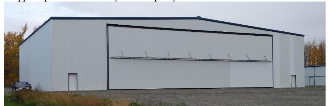
(Photo: Aurora Sky LLC hangar is 100' X 120' with an 80' wide Schweiss bifold door with 22' clearance)
