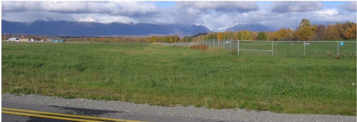
Figure 6: Golf Course Fence in Runway Object-Free Area
