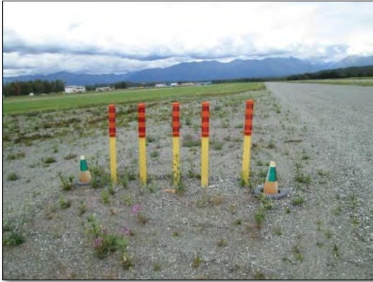
Figure 2-8. Runway 16S-34S Threshold Markers
