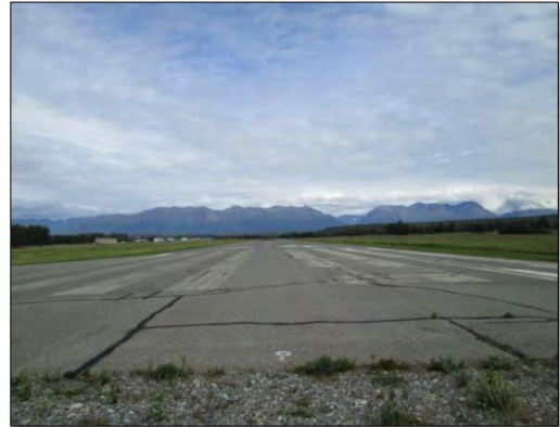
Figure 2-5. South Section of Runway 16-34
