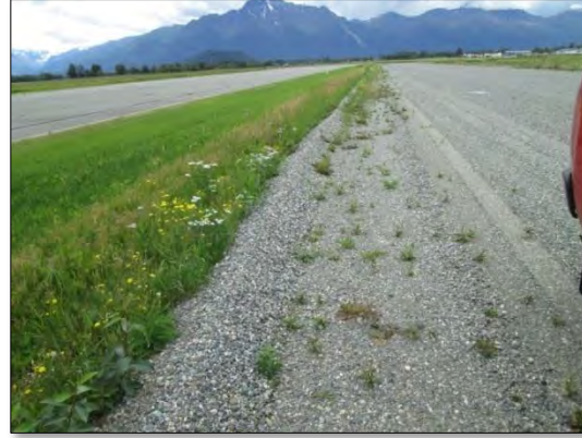
Figure 2-9. Runway 16S-34S Gravel Berm
