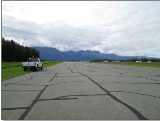
Figure 2-4. North 500 feet of Runway 16-34 (Displaced Threshold Area)
