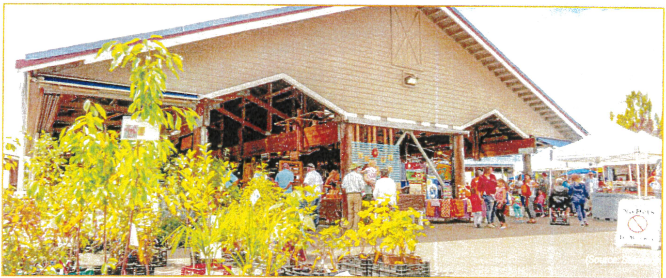
Above: Example of a public Farmer's Market building (Olympia, WA)
