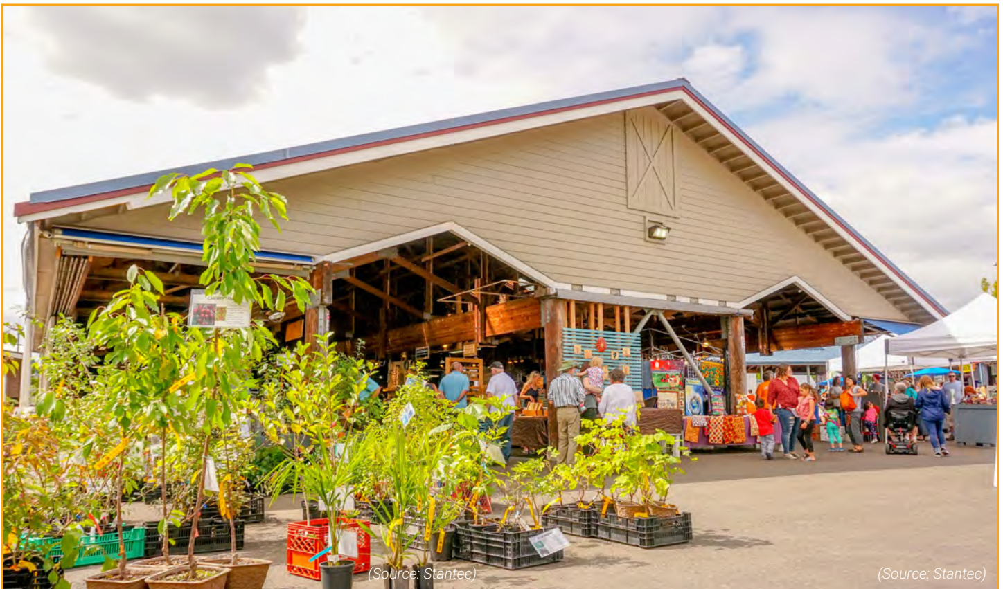
Top: Example of a public Farmer’s Market building (Olympia, WA)
