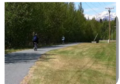
Cope Industrial Way Bike Path
