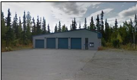
Station 3-5 8200 E. Turner Rd. Calls for Service – 133
