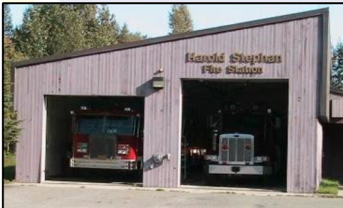
Station 3-2 5955 N. Glenn Hwy Calls for Service – 58
