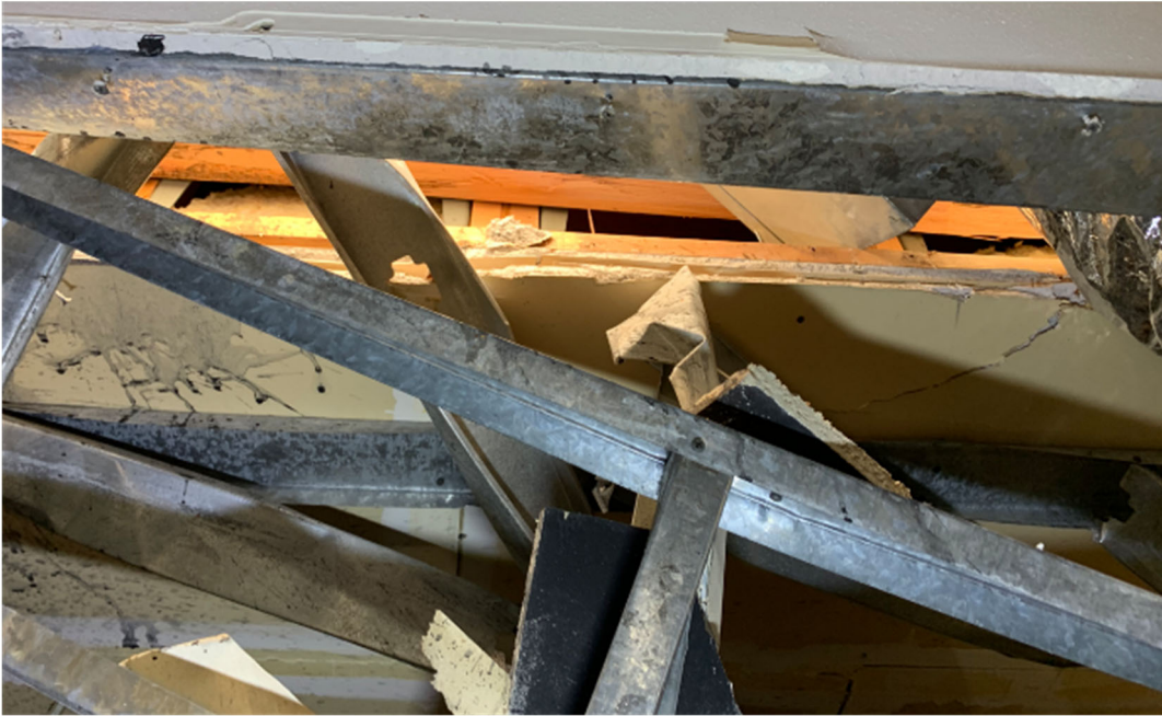
Photo 8: Joist in Top Flange Hangers
