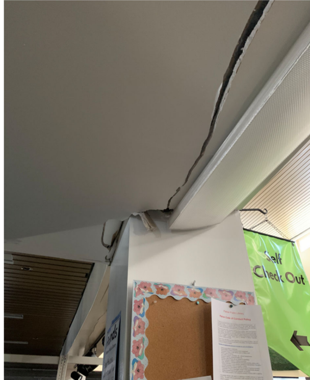
Photo 6: Crushed Soffit
