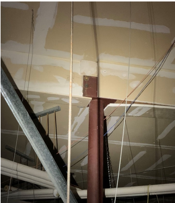
Photo 4: Beam Centered Over Column
