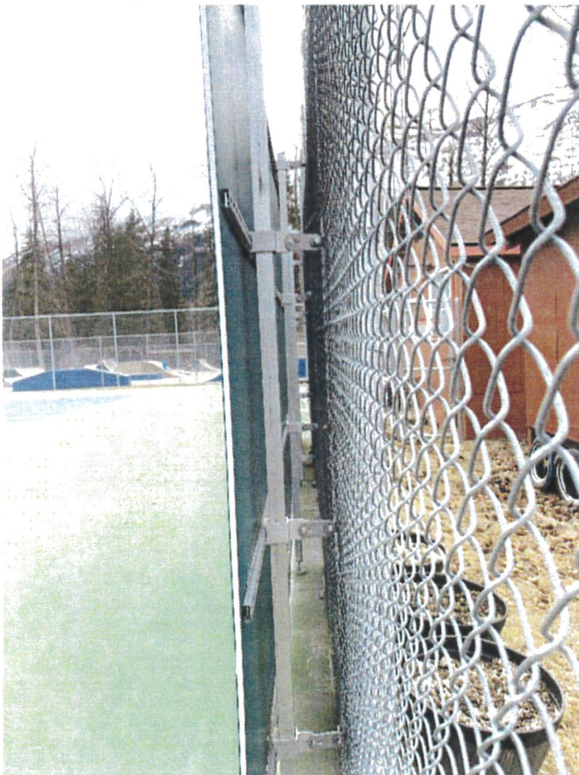
Rally Master Back Board fence post connection
