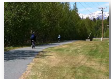
Cope Industrial Way Bike Path
