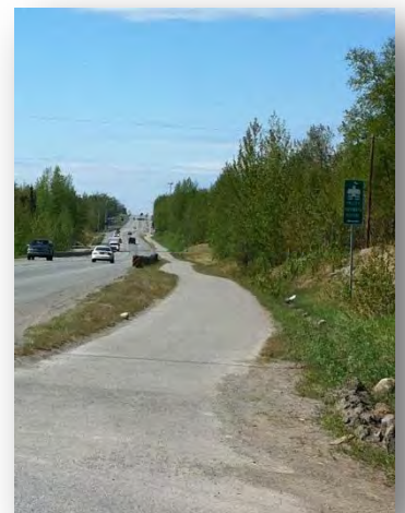
Paved trail along Palmer-Wasilla Highway
