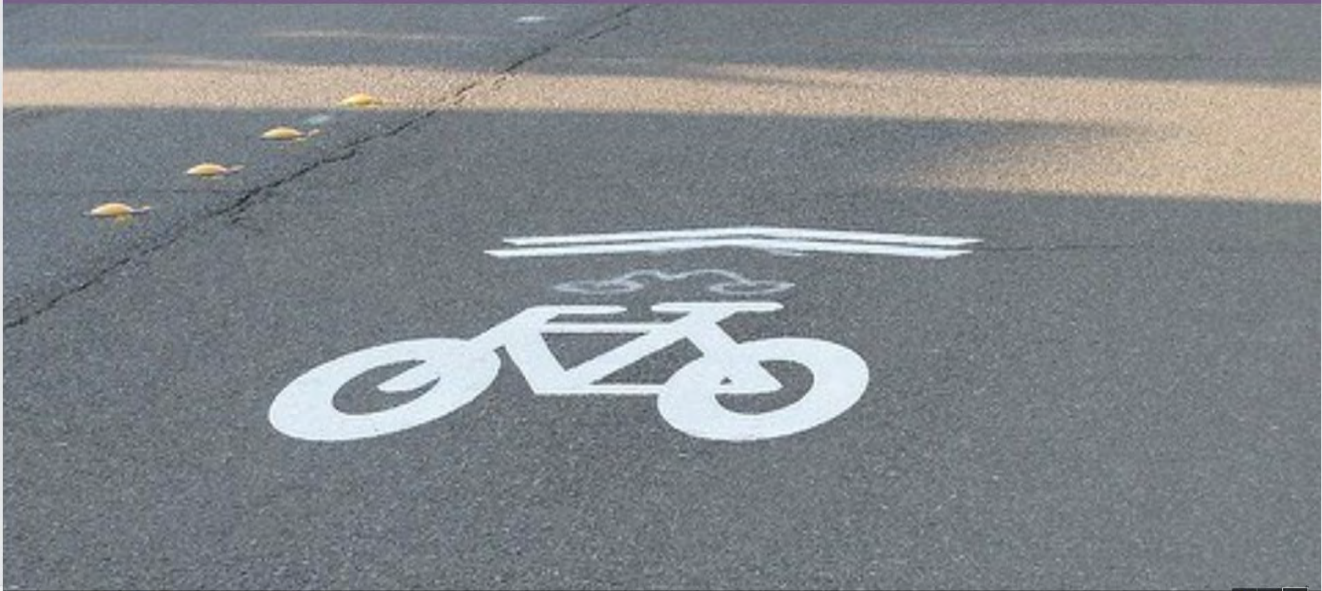
Label lanes so it's clear to all that it is a mixed use road
