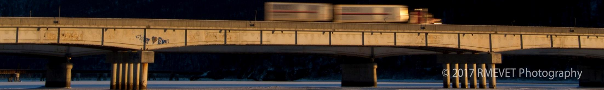
Knik River Bridge
