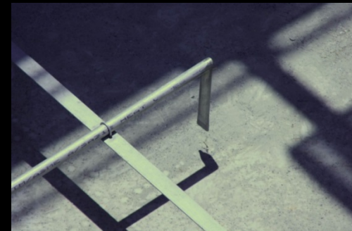
MBBR Coarse Bubble Diffusers
