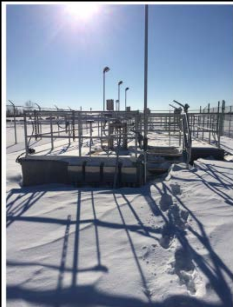
Cold Weather (-21°F) MBBR installation in Wisconsin
