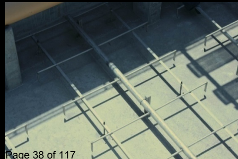
MBBR Coarse Bubble Diffusers
