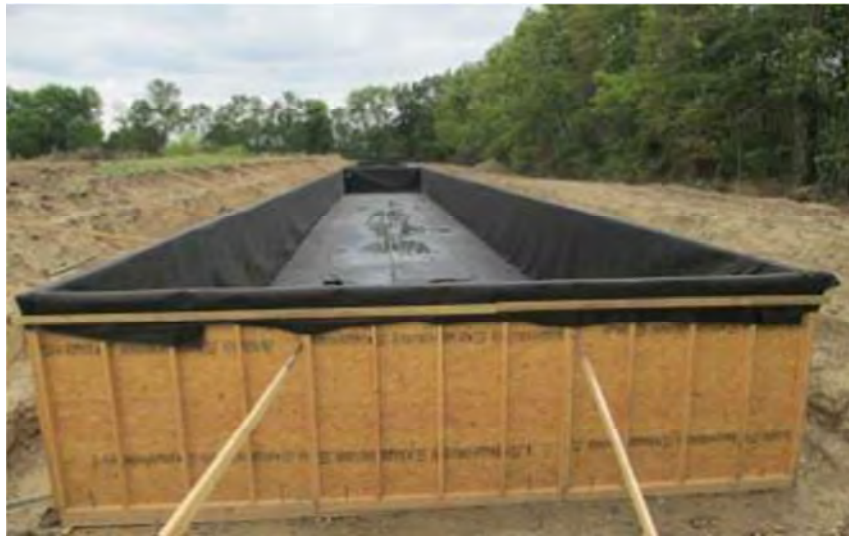
Figure 20 Photos of SAGR Installation
