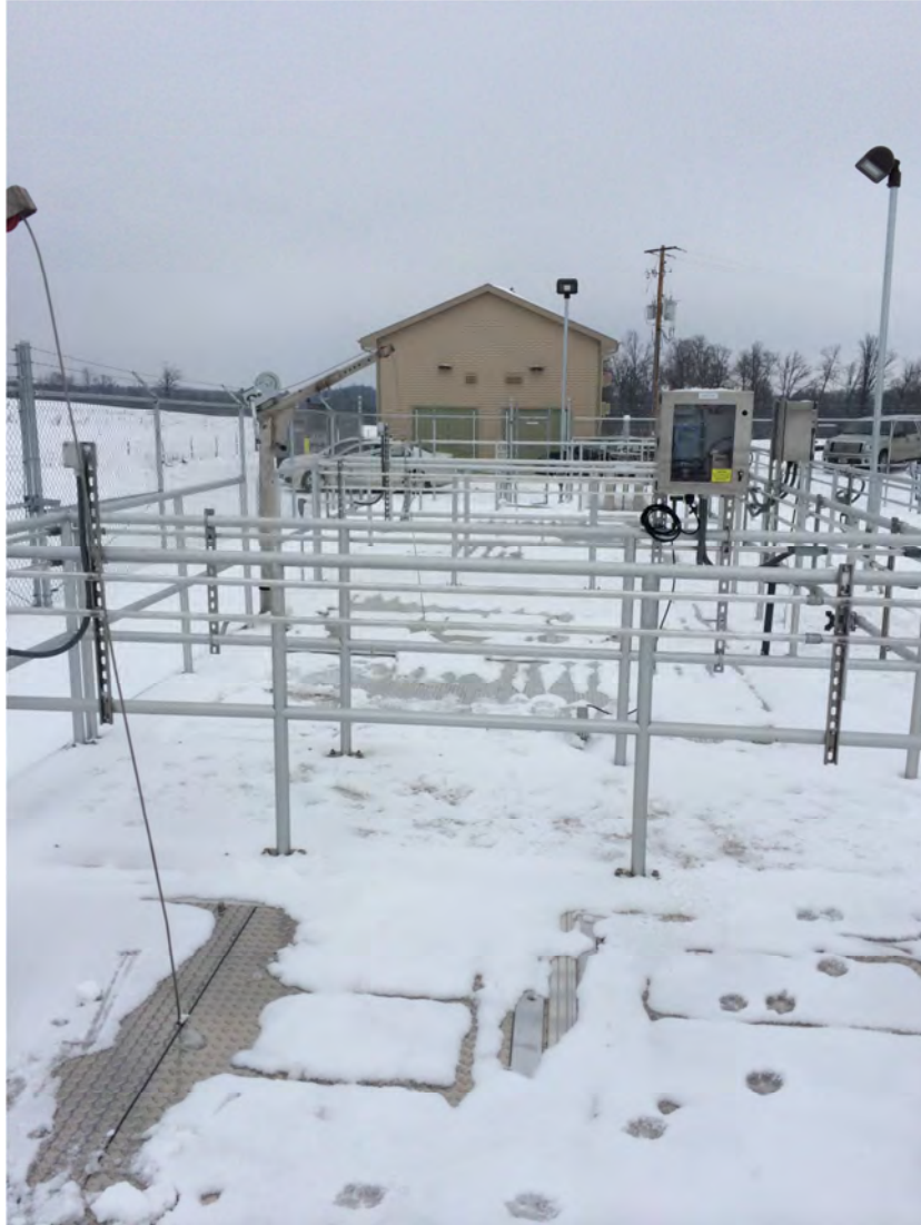
Figure 33: Cold Weather (-21F) MBBR Installation in Wisconsin
