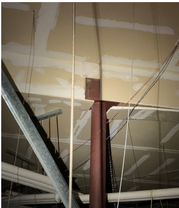
Photo 4: Beam Centered Over Column
