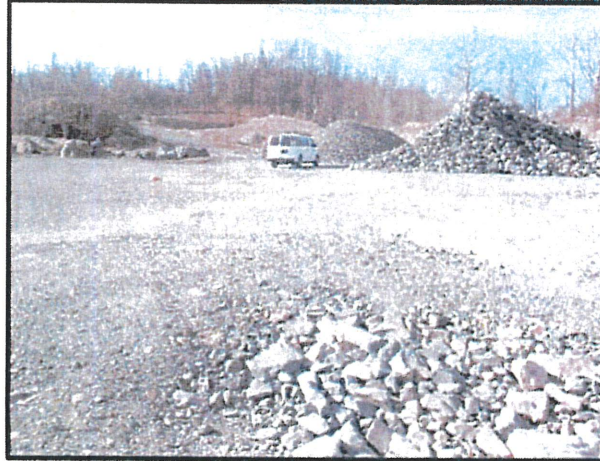
Photo 1 – Project Site Surface Conditions Viewing south-southwest from approximate NE site corner
