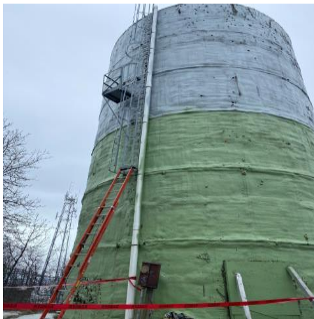
Figure 4: In-use overflow pipe
