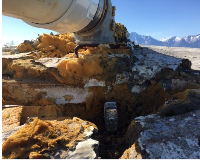
Figure 8: Overflow roof connection
