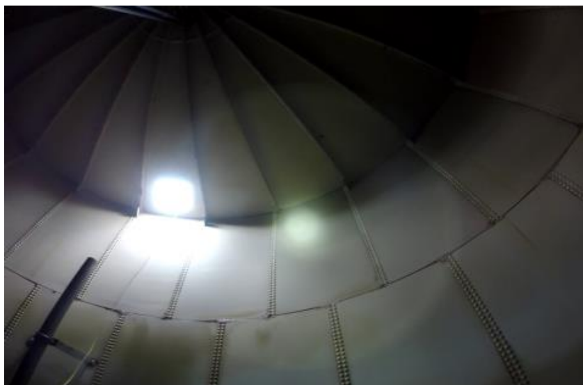
Figure 20: Roof with walls visible
