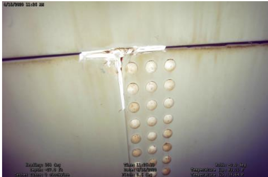
Figure 15: Example of caulking in seams
