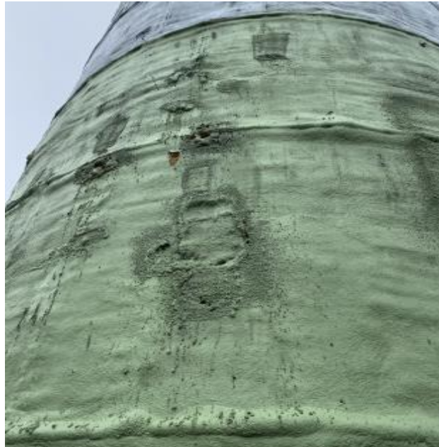
Figure 2: Insulation deterioration
