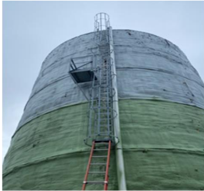
Figure 6: Access ladder and balcony
