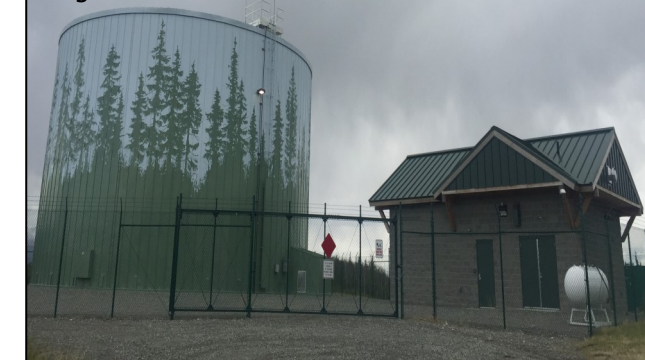
Reservoir # 4 off Trunk Rd holds 1 million gallons of water.
