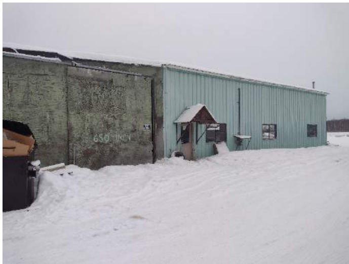
Photo 1. Building Exterior (Facing East)
