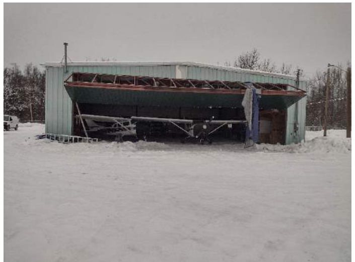
Photo 2. Building Exterior (Facing North)
