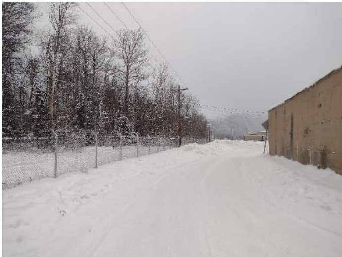
Photo 15. Building Transformer (Facing East)
