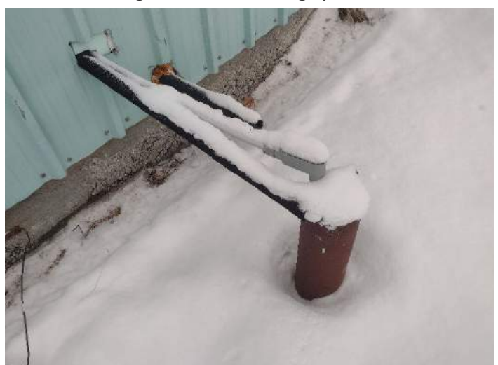
Photo 6. Water Supply Well and Sink Drainage
