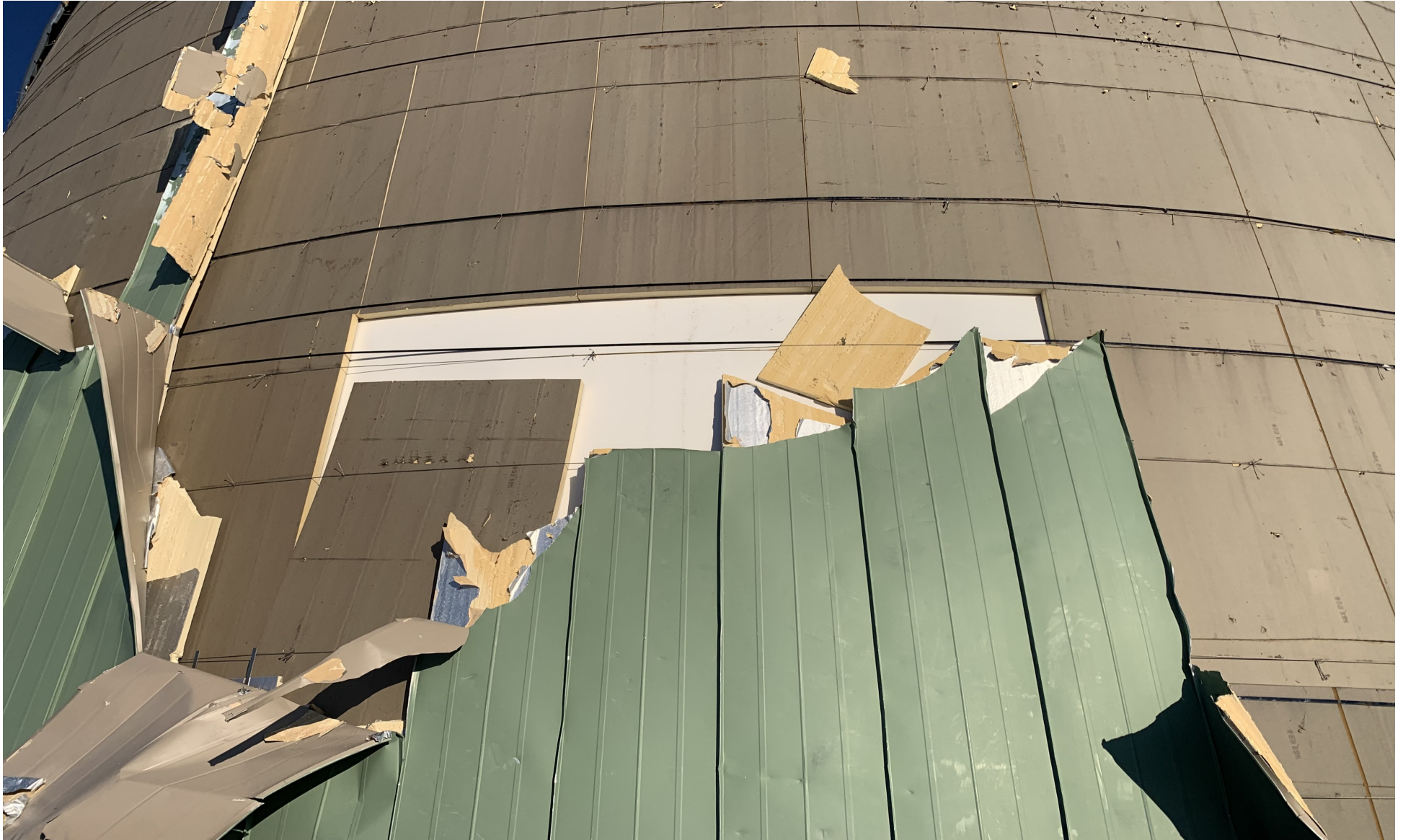
Palmer Reservoir 4 - Photo 2 of 4: Damage to Siding and Insulation Layers showing exposed tank shell (white)
