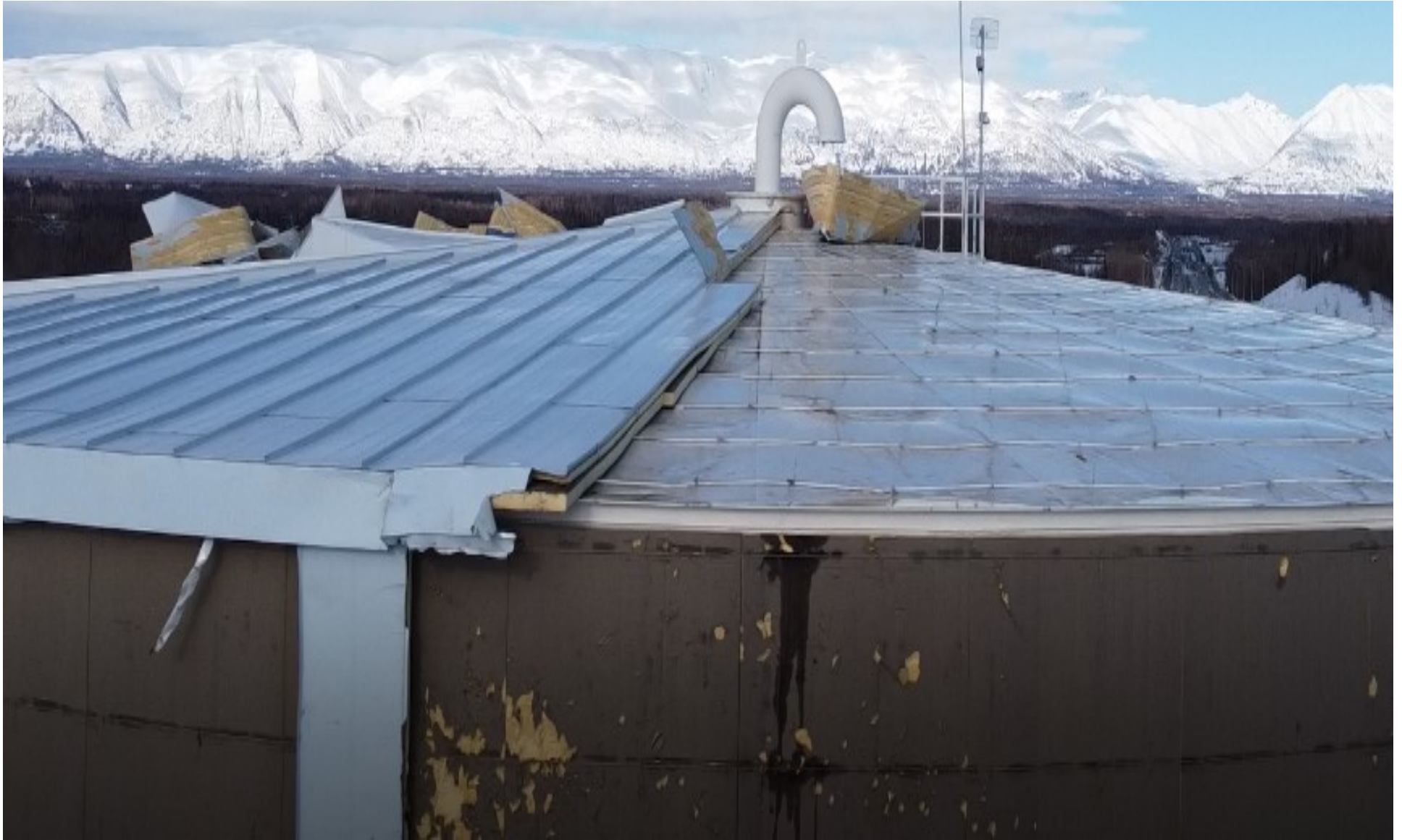
Palmer Reservoir 4 - Photo 3 of 4: Drone View of Roof Damage
