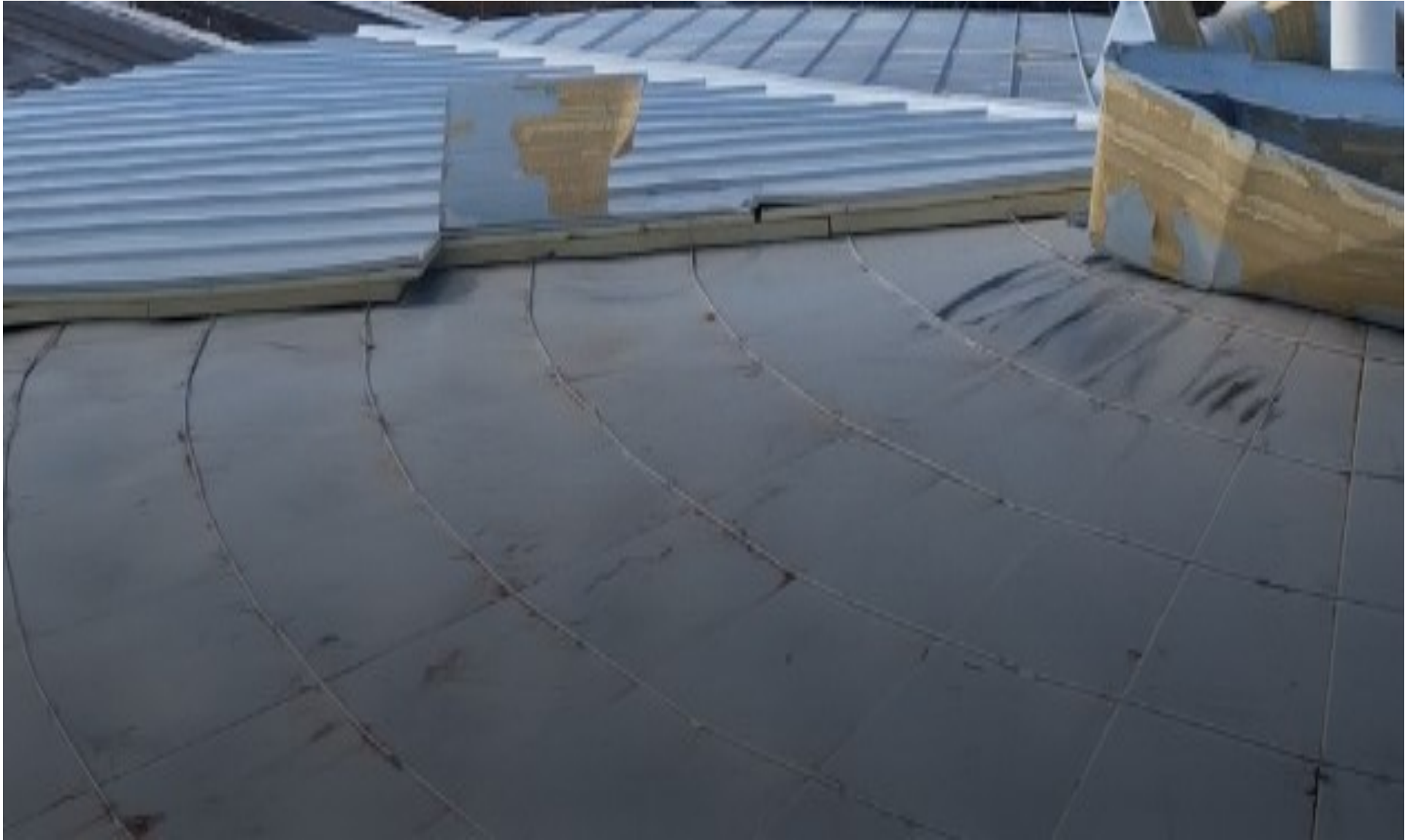
Palmer Reservoir 4 - Photo 4 of 4: Drone View of Roof Damage showing Grid Rods, Insulation Layers, and Galvalume Sheathing
