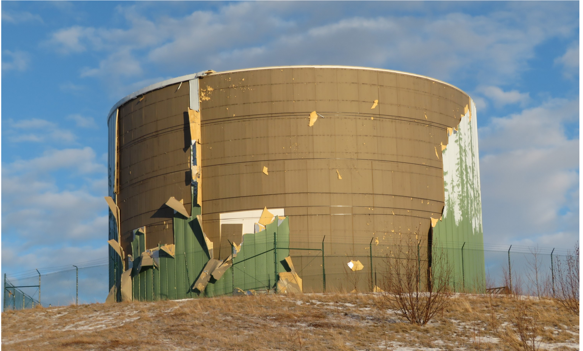
Palmer Reservoir 4 - Photo 1 of 4: Ground View of Damage to Siding and Insulation Layers
